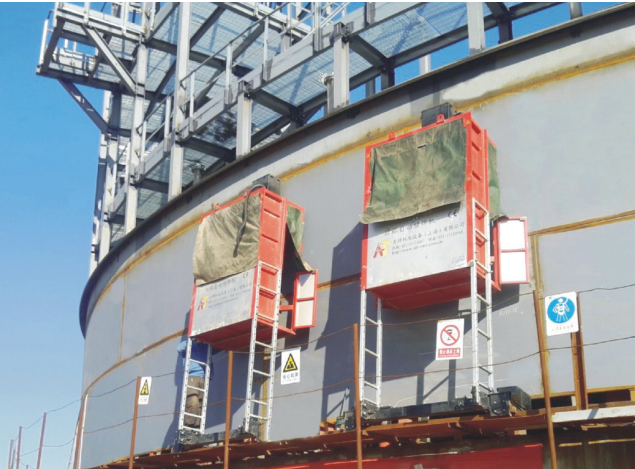
大型贮槽自动横焊机 Large-sized Storage Tank Automatic Girth Welding Machine
