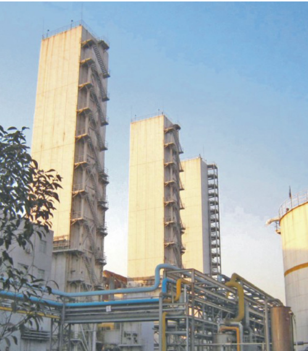
邯钢 2X35000Nm 3 /h 稀有气体全提取空分设备 Handan Iron and Steel 2X35000Nm 3 /h rare gas full extraction air separation plant
