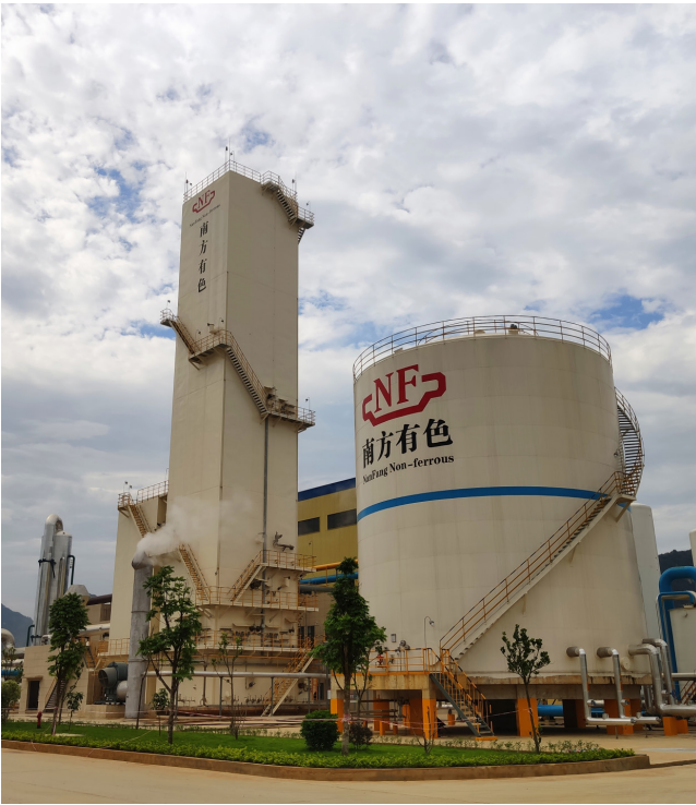
广西南国 42000Nm 3 /h 低纯富氧新型空分 Guangxi Nanguo 42000Nm 3 /h low-purity oxygen-enriched new air separation
